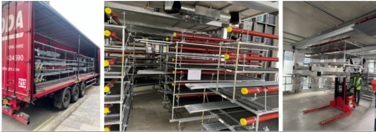
4 M&E racks, being delivered to site and installed. ©Bryden Wood.
