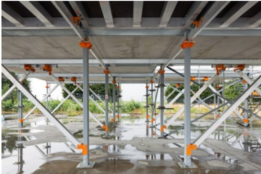
1 MoJ Platform 2, with temporary works in place. ©Bryden Wood.
