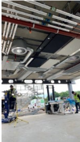
3 M&E installation being tested on the prototype. ©Bryden Wood.
