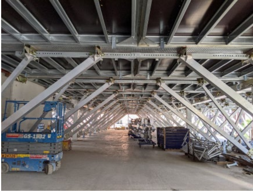
2 Landsec Platform, also with temporary works in place. ©Bryden Wood.
