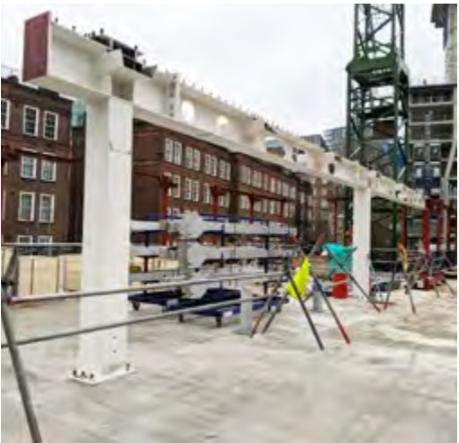
Long-span beam in place at The Forge.
