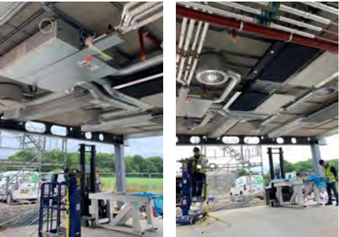
Installation of prototype M+E cassettes.
