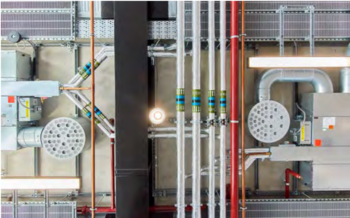
MEP attached to fixing points cast into the soffit.
