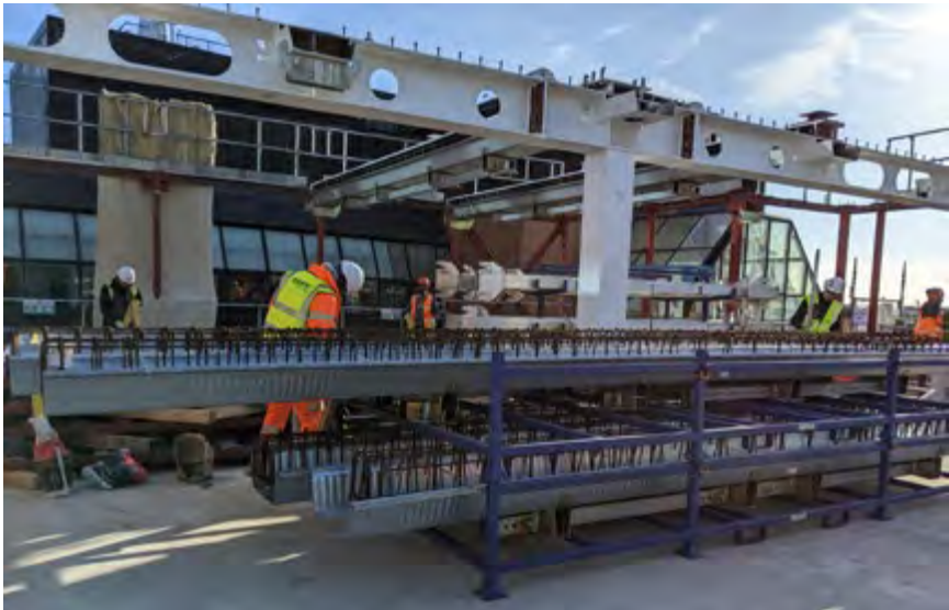
Stillage containing multiple beam shutters with reinforcement cages pre-installed at The Forge.
