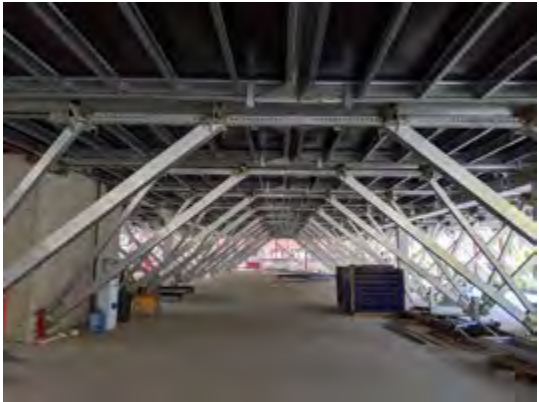
Temporary props in place at The Forge.
