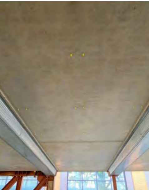
Completed soffit on-site. Note fixing points for MEP cast into slab
