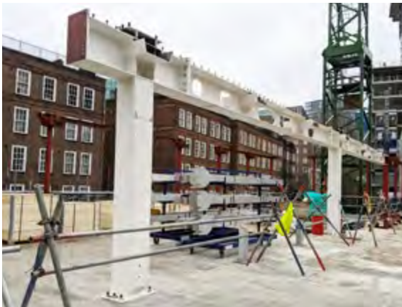
Long-span beam with overprovision of penetrations for future MEP adaptability.
