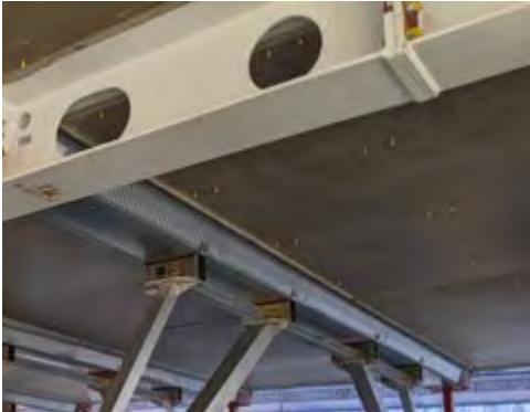
4. Completed slab soffit, with MEP fixing points visible.
